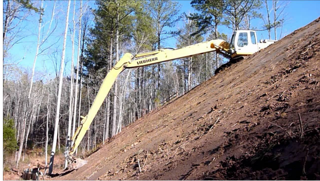
Excavator grading a slope (source: www.youtube.com/watch?v=FM5w5xOZqn0 )
