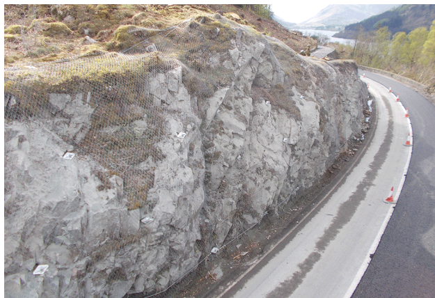
Rock bolting and netting used to support a cliff in Thirlmere, Cumbria (Source: www.can.ltd.uk/ )
